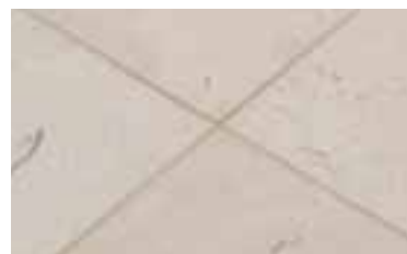
Moisture sensitive natural stones grouted with ARDEX MG rapid drying marble and natural stone grout. ARDEX 'Rapidry Formula' technology locks the mix water into the grout, eliminating water staining at the tile edges.
