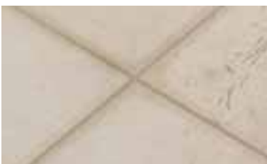
Moisture sensitive natural stones grouted with a traditional cement-based grout, resulting in unsightly water staining at the tile edges.
